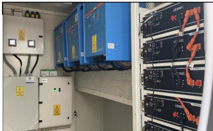
Figure 6 Battery packages (right) and battery inverter (left)
